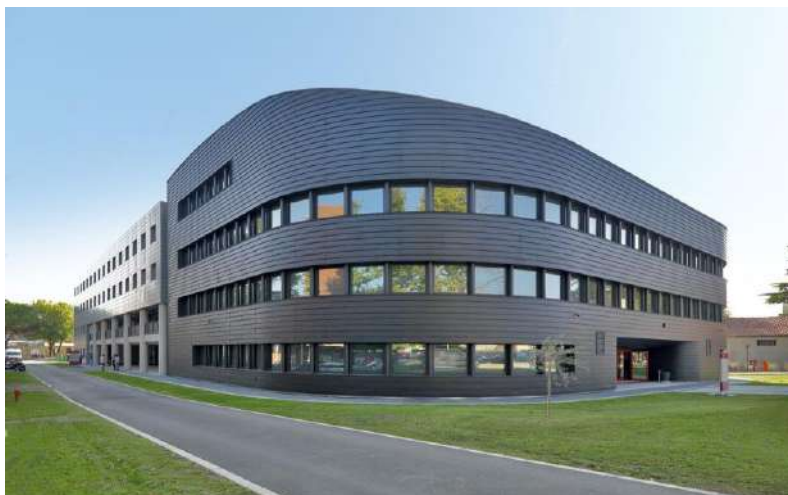
Figure 3. Exterior metal cladding application
