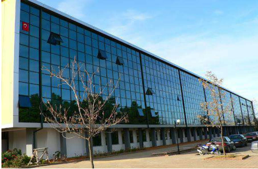
Figure 11. An application where silicone and glass are used together on the exterior
