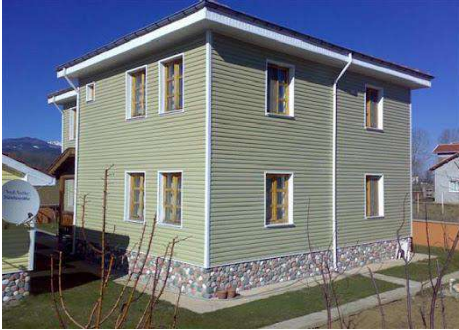
Figure 13. PVC-Siding application on exterior
