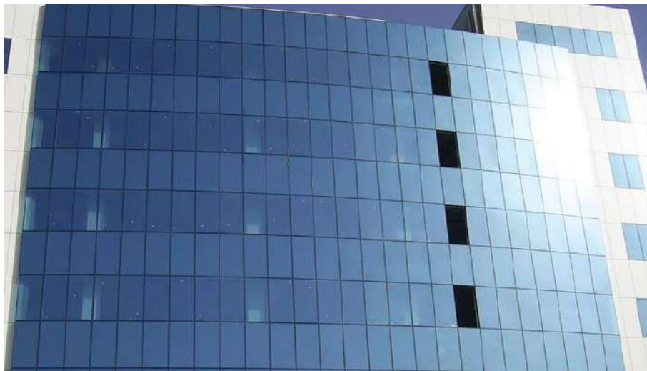
Figure 12. Facade application where composite-silicone and glass are used together on the exterior
