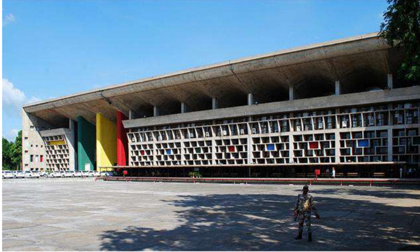
Figure 19. High Court Chandigarh-india-1951
