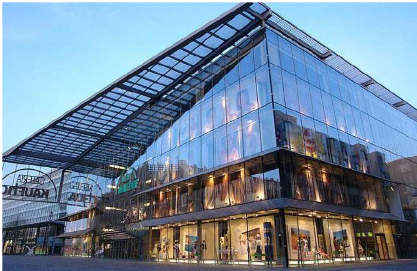
Figure 7. Exterior glass application
