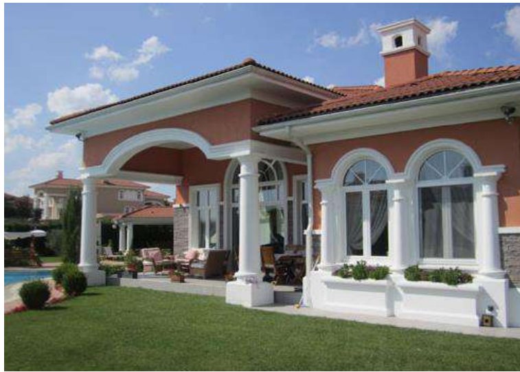
Figure 1. Precast application on exterior
