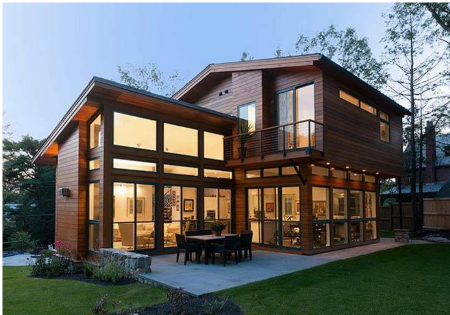
Figure14. Exterior wood application
