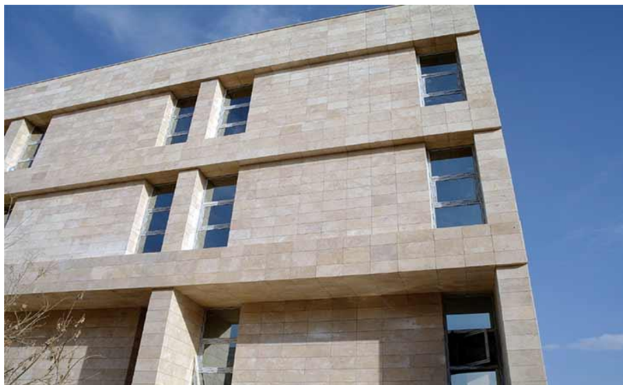
Figure 9. Marble application on the exterior
