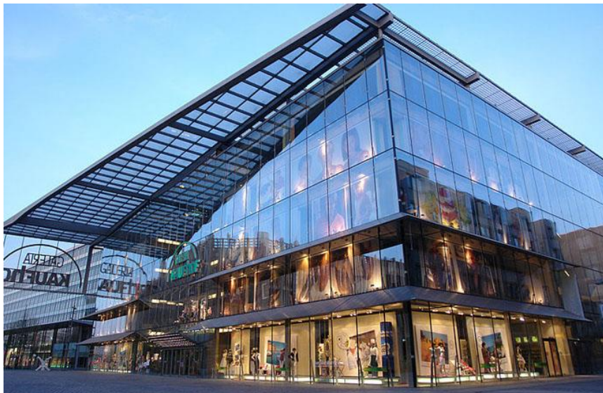
Figure 7. Exterior glass application
