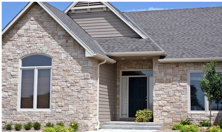
Figure 2. Stone application on the exterior
