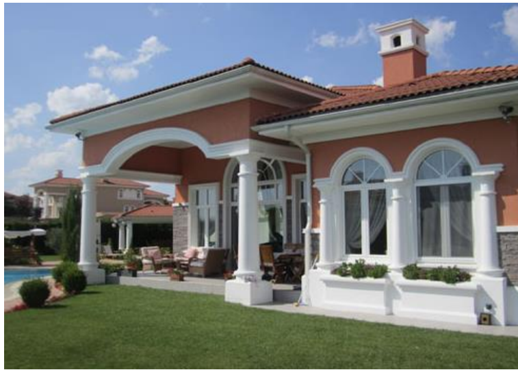
Figure 1. Precast application on exterior
