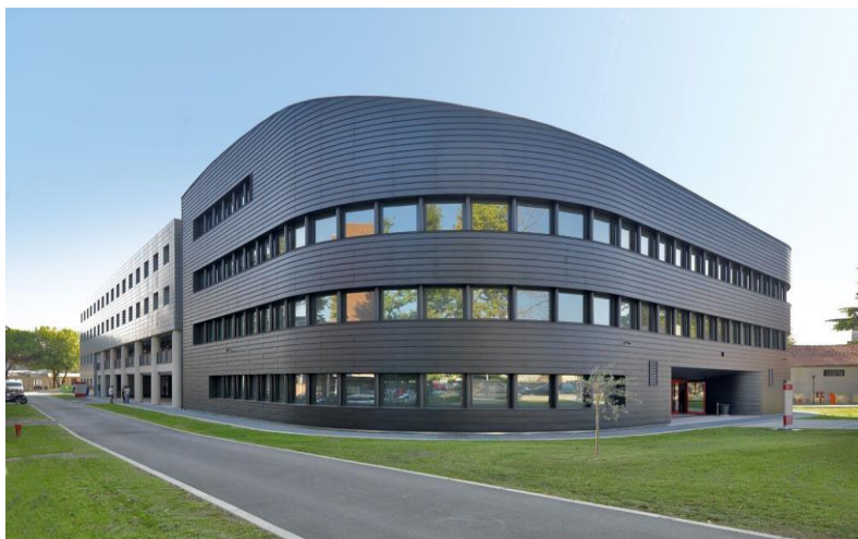
Figure 3. Exterior metal cladding application
