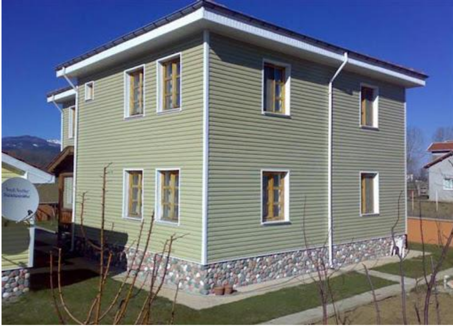
Figure 13. PVC-Siding application on exterior
