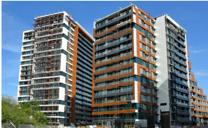
Figure 6. Buildings with exterior composite application
