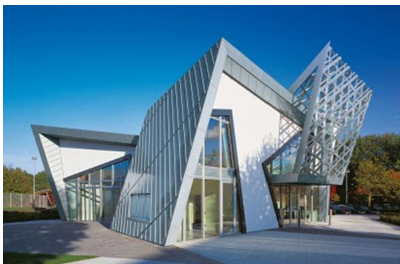
Figure 4. Modern metal cladding application on the exterior
